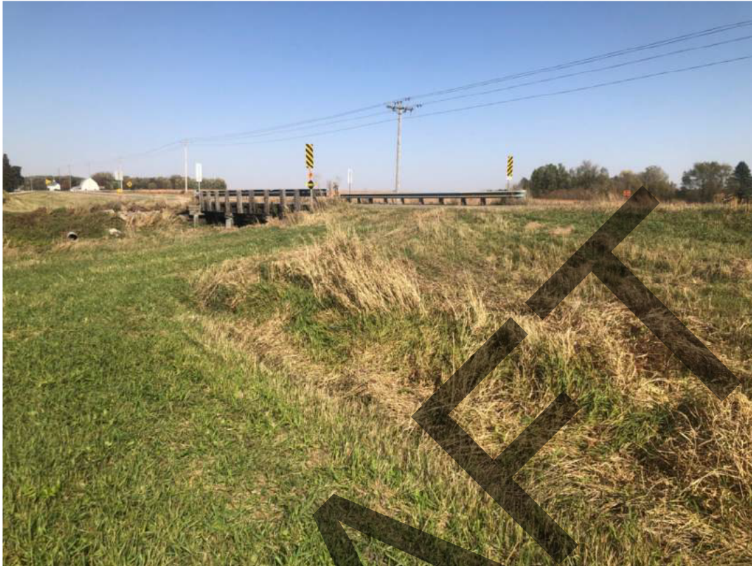
Photo 2.1 – Field driveway south of Bridge 74519, looking northeast
